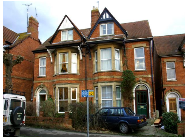
© Nigel Andrews 2002 SSDC ENVIRONMENTAL HEALTH BEDSIT CONVERSION FEATURES 240 U2802: a typical semi-detached residence suitable for conversion into bedsit accommodation. Photo by: Nigel Andrews
